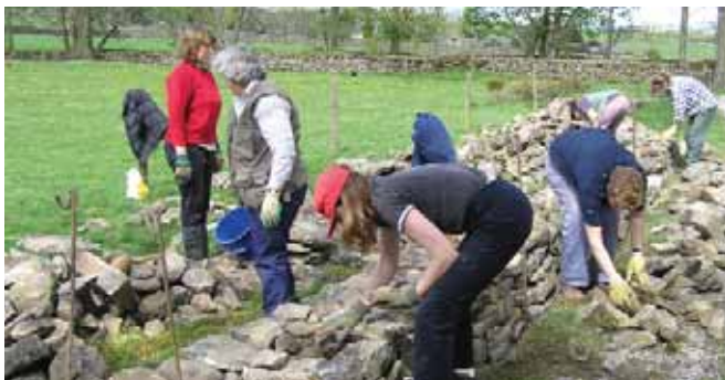
Repairing the drystone walling
